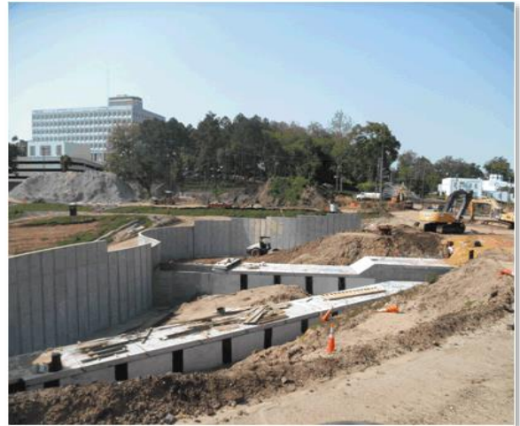
Figure 8. Redevelopment work at the site.
