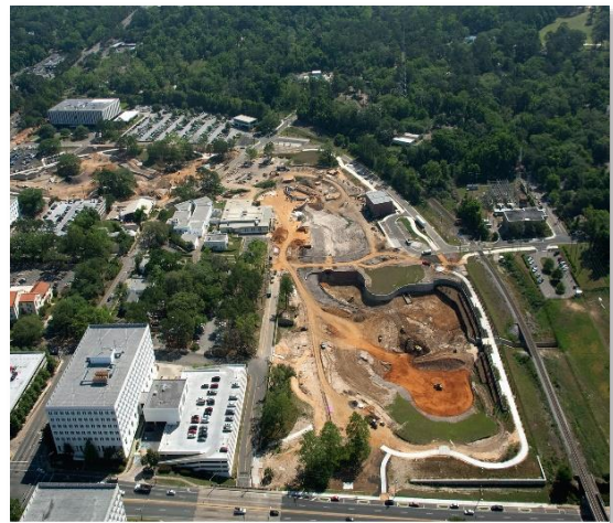
Figure 4. Aerial view of Cascades Park during construction.
