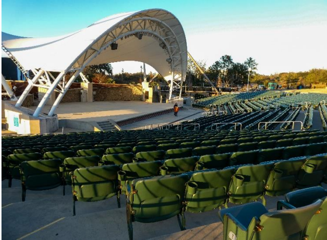
Figure 12. The Adderley Amphitheater with its 3,240 seats during the day.
