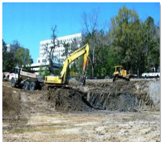
Figure 7. Excavation as part of environmental cleanup at the site.
