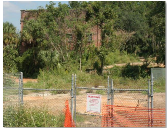
Figure 5. Security fencing and warning signs at the site in 2006.
