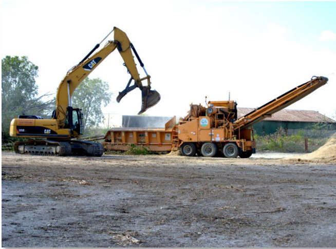
Figure 7. Crews preparing the site for solar project installation.
