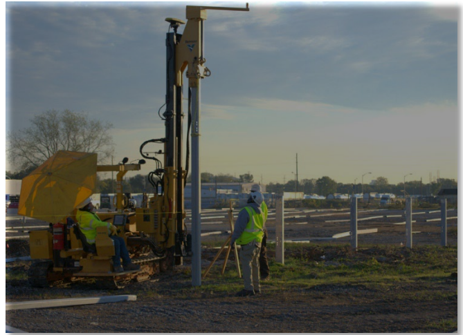
Figure 8. A driven-pile method was used in place of concrete ballasts.
