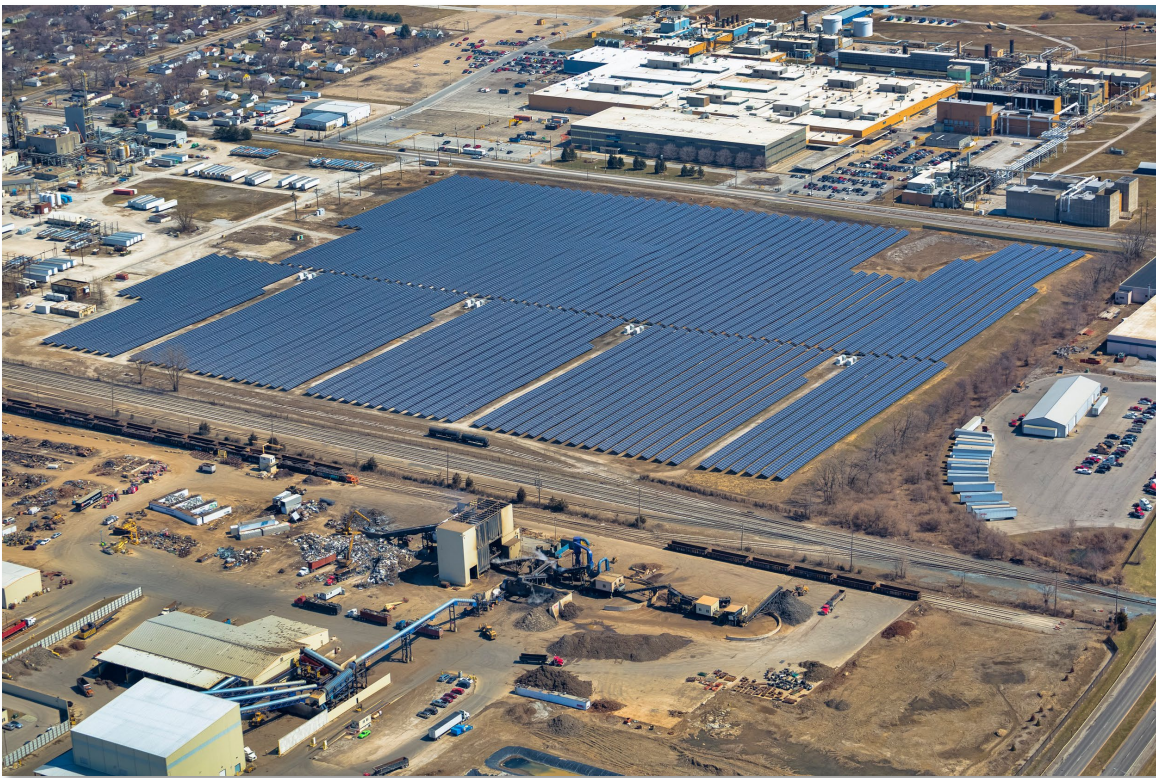
Figure 13. An aerial view of Maywood Solar Farm.
