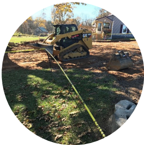
Residential yard during excavation.
