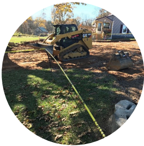
Residential yard during excavation.
