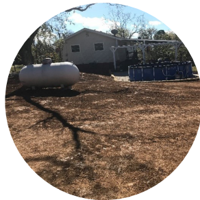
Residential yard backfilled with clean soil.
