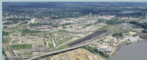
The former ASARCO facility property after demolition.
