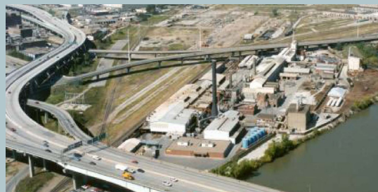
Aerial view of the former ASARCO facility prior to demolition in 1997.
