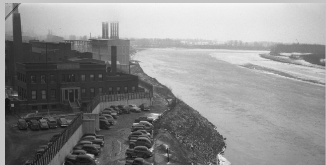
Installation of flood walls helped protect the ASARCO facility from flooding. Image from the Omaha World-Herald/John Savage Photography Collection at The Durham Museum, used with permission.
