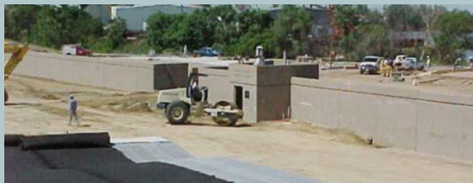
Placement of a liner system to contain lead-contaminated soils in a "burrito" prior to adding several feet of clean soil as a cap.
