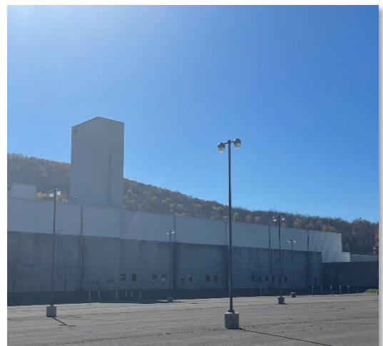
Figure 9. View of the renovated former factory building at the site, now a document storage warehouse.
