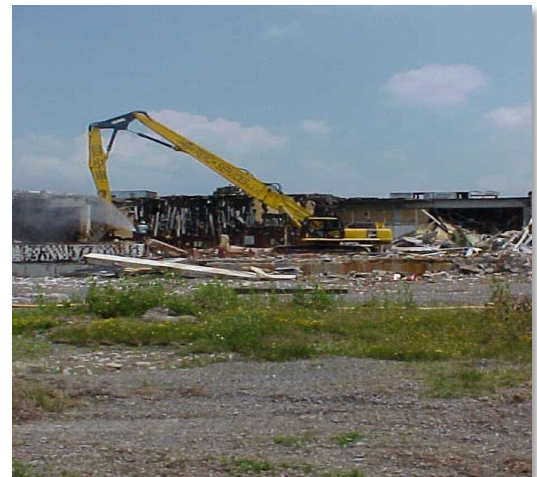
Figure 3. Cleanup required demolishing structurally damaged and contaminated buildings.
