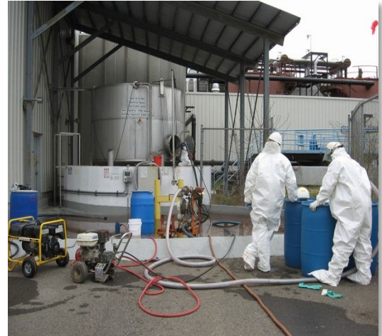
Figure 2. Workers cleaning up hazardous materials on site in the late 2000s.
