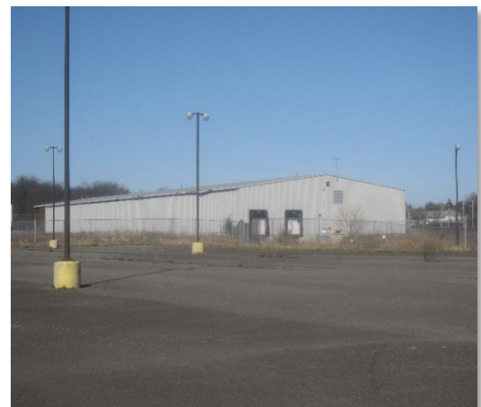
Figure 4. The warehouse on site, prior to its renovation for Bio365 operations.
