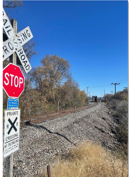
Figure 10. Rail access at the Cortland Industrial Center.
