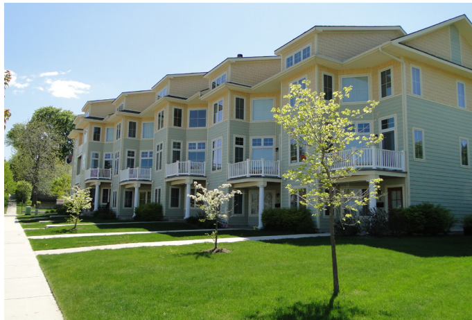
Figure 7. Townhomes at the PMC Groundwater site (Michigan).
