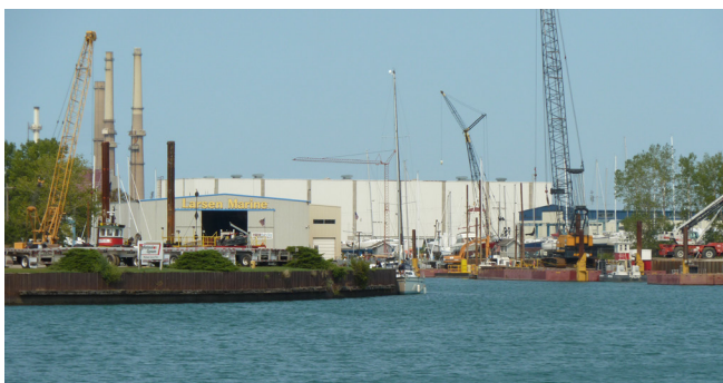
Figure 25. Cranes along the Waukegan Marina support industrial businesses at the Outboard Marine Corp. site (Illinois).
