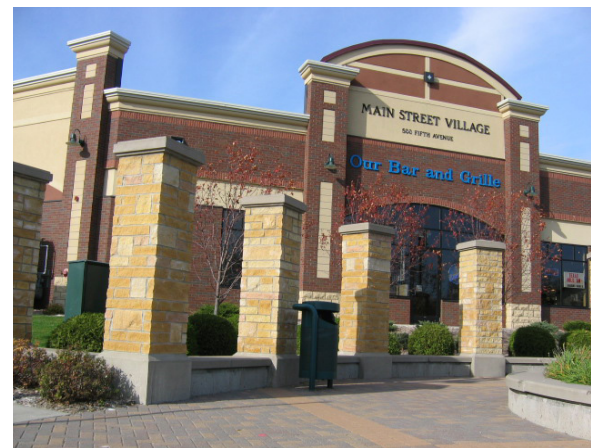
Figure 16. A restaurant at New Brighton Corporate Park III at the MacGillis & Gibbs Co./Bell Lumber & Pole Co. site (Minnesota).
