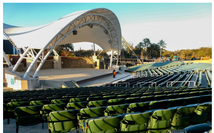
Figure 10. The Capital City Amphitheater at Cascade Park at the Cascade Park Gasification Plant site (Florida).
