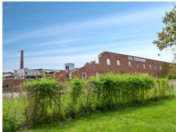
Figure 23. The former textile facility at the US Finishing/Cone Mills site (South Carolina).
