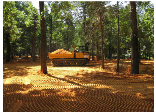
Figure 17. As part of cleanup, a sand cover was put in place to protect habitat at the Ciba-Geigy Corp. (McIntosh Plant) site (Alabama).
