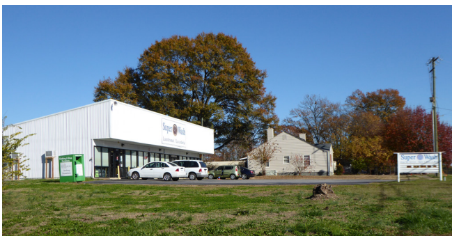
Figure 31. Industrial and commercial uses at the Elmore Waste Disposal site (South Carolina).
