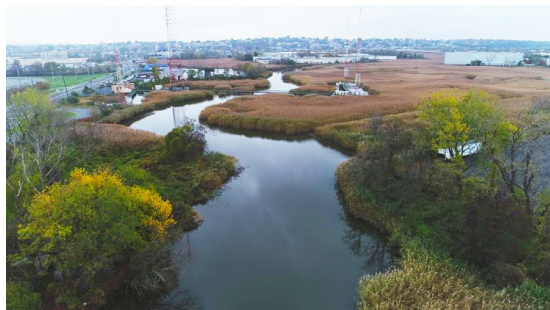
Figure 18: Top: Warehouse loading bays on the Ventron/Velsicol site (New Jersey). Bottom: Aerial View of Berry's Creek near the Ventron/Velsicol site (New Jersey).
