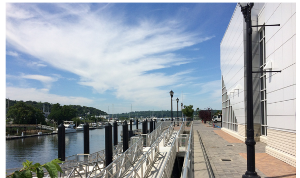
Figure 17: Top: The Glen Cove Ferry Terminal office at the Li Tungsten Corp. site (New York). Bottom: The esplanade walkways along the Glen Cove Ferry Terminal dock at the Li Tungsten Corp. site (New York).
