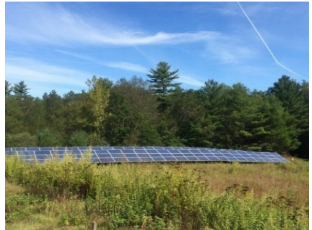
Figure 84. Solar panels are used to power the groundwater treatment system at the Re-Solve, Inc. site (Massachusetts).
