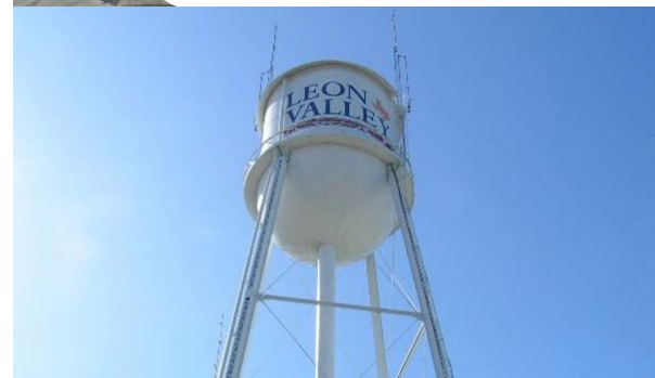
Figure 3. Leon Valley Municipal Water Supply tower
