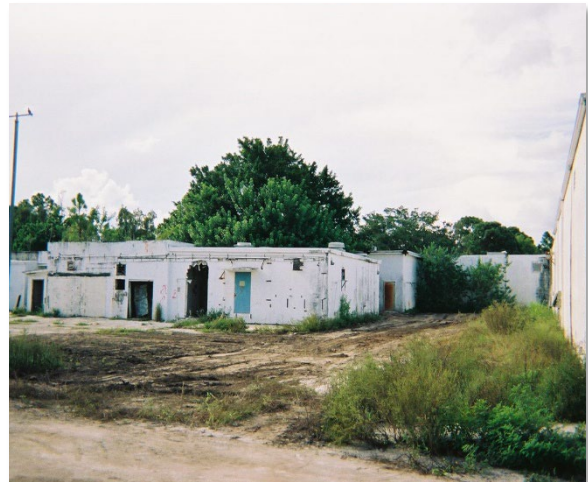
Figure 3. Site buildings before cleanup and construction.
