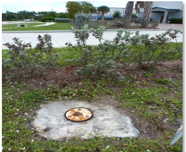
Figure 5. A groundwater monitoring well is integrated into landscaping near a new warehouse.
