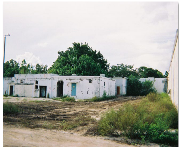
Figure 3. Site buildings before cleanup and construction.
