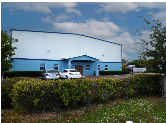
Figure 10. The warehouse on Lot 5 where three businesses operate.
