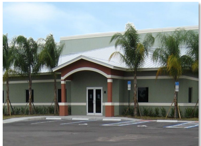
Figure 11. Front of the Stuart Web, Inc. warehouse.
