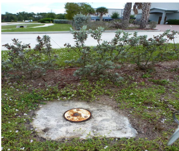
Figure 5. A groundwater monitoring well is integrated into landscaping near a new warehouse.
