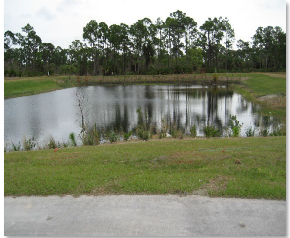
Figure 4. The stormwater retention pond located on site.
