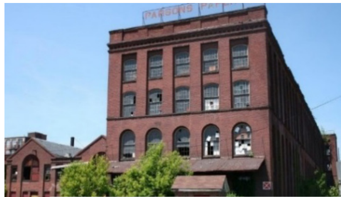
Figure 3. Former mill building before demolition
