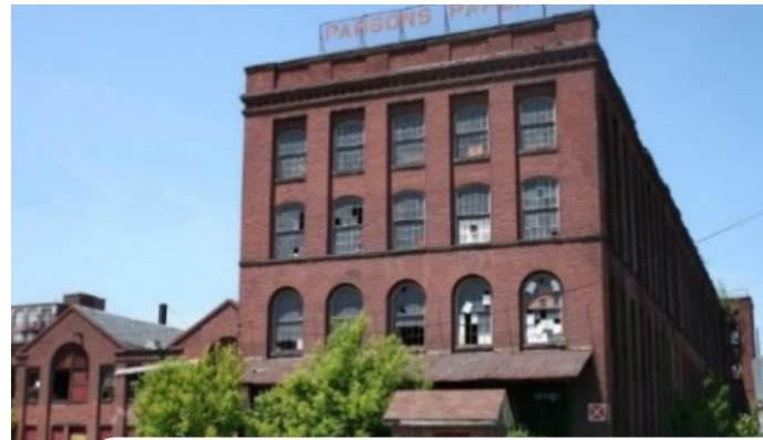
Figure 3. Former mill building before demolition
