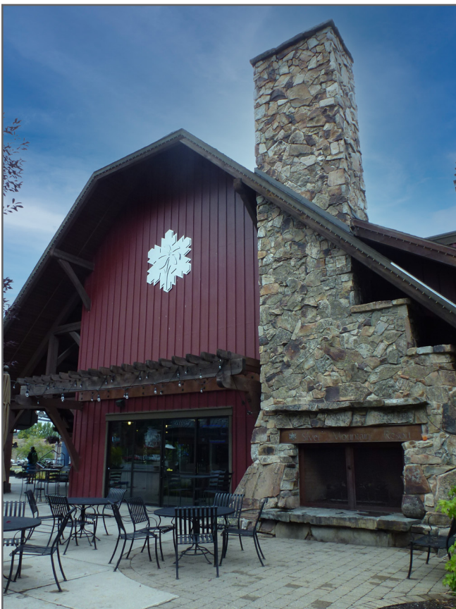
Restaurant at the Bunker Hill Mining & Metallurgical Complex Superfund site in Smelterville, Idaho.
