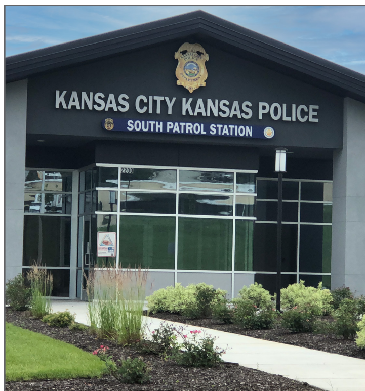
Police Station at the Kansas City Structural Steel Superfund site in Kansas City, Kansas.
