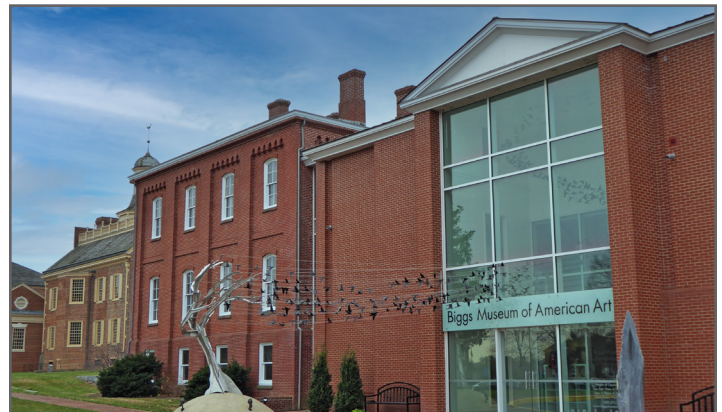
Museum at the Dover Gas Light Co. Superfund site in Dover, Delaware.
