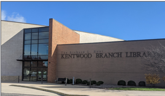
Library at the Kentwood Landfill Superfund site in Kentwood, Michigan.
