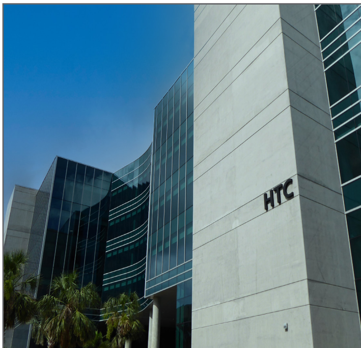
Harris Technology Center at the Harris Corp. (Palm Bay Plant) Superfund site in Palm Bay, Florida.
