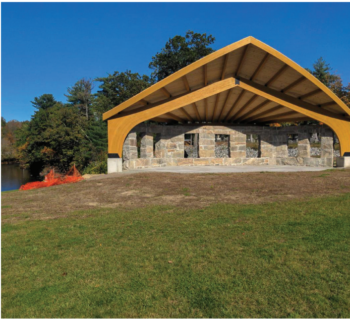
Figure 8. A view of the Korean War Memorial and recreational space at the Fletcher's Paint Works and Storage site (New Hampshire, Region 1).
