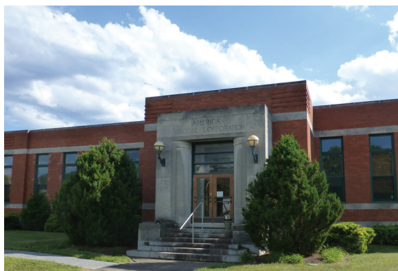
Figure 15. The former American Viscose Corporation administrative building at the Avtex Fibers site has been refurbished and now hosts several small businesses (Virginia, Region 3).
