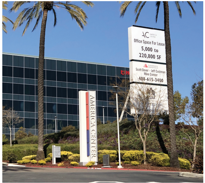
Figure 9. America Center at the South Bay Asbestos site (California, Region 9).
