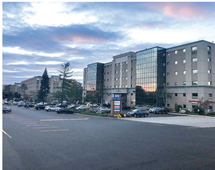
Figure 11. Businesses that are part of the mix of commercial, industrial and residential areas at the Wells G&H site (Massachusetts, Region 1).
