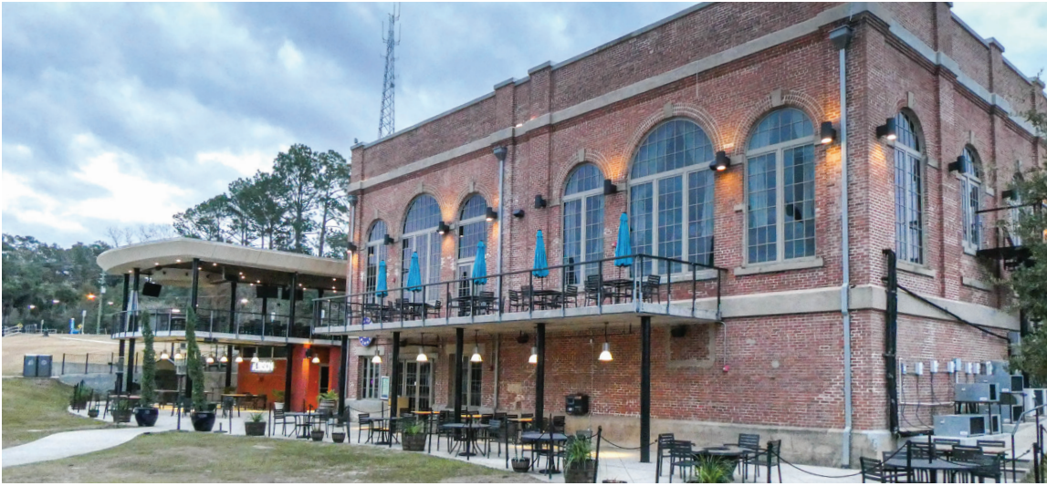
Figure 1. Two businesses operate at the Cascade Park Gasification Plant site (Florida, Region 4).
