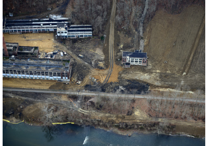
Aerial view of the site prior to cleanup.
