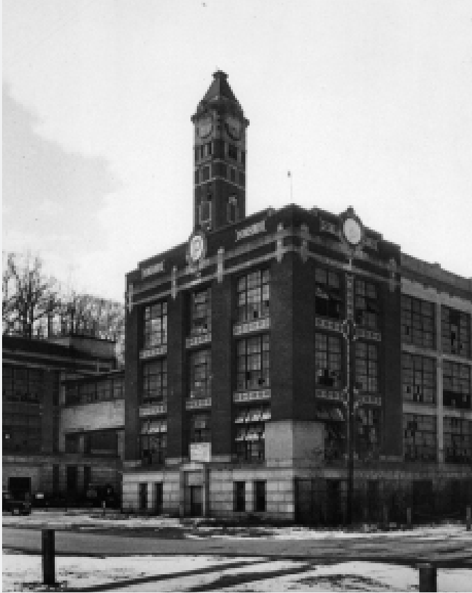
Clocktower and factory buildings at the site.
