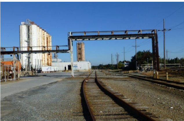
Figure 2. PVC plant prior to demolition.
