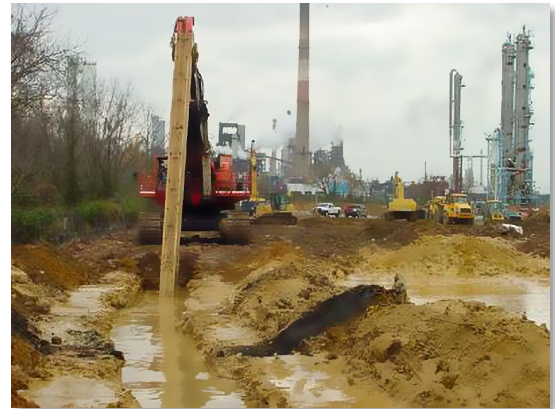
Figure 4. Delaware City PVC Plant Site during cleanup.
