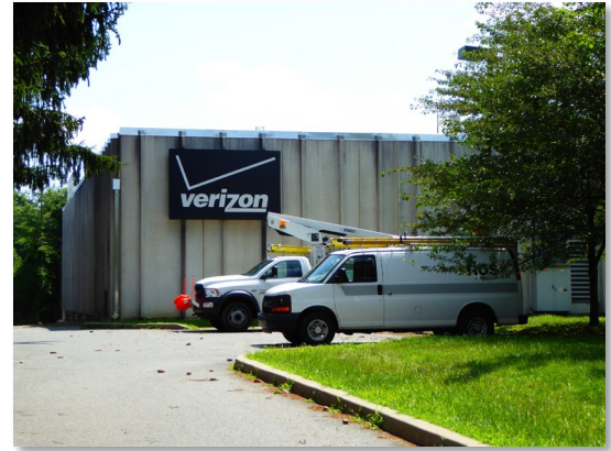
Figure 8. Verizon telecommunications utility service center on the southern edge of the Site.
