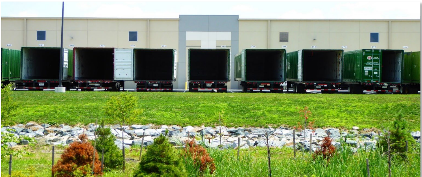
Figure 12. View of Dart Container's loading area.
