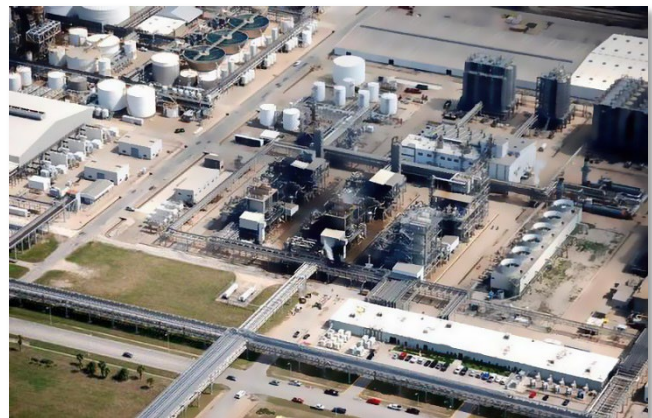
Figure 3. Aerial view of PVC plant prior to demolition.
