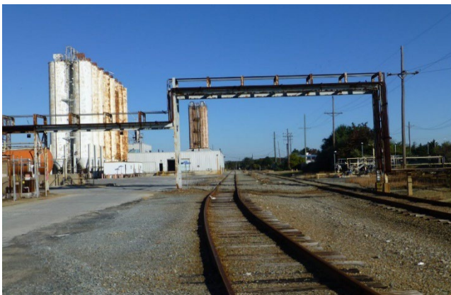
Figure 2. PVC plant prior to demolition.
