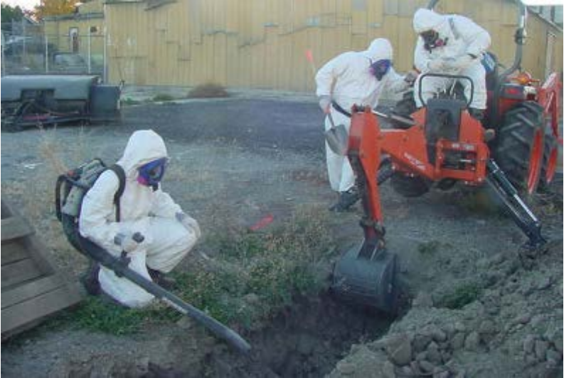
Checking a trench area.
