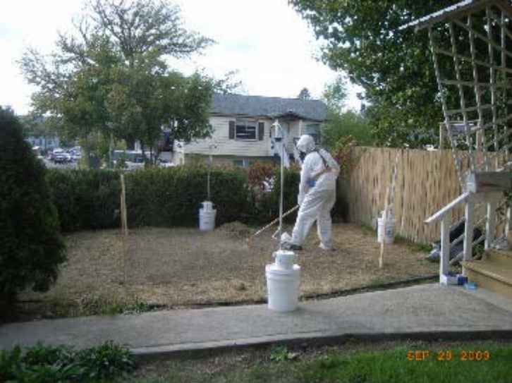
Raking scenario with perimeter monitoring.
