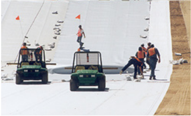
Figure 9: Remedial workers placing a liner system at base of disposal cell (left). The placement of the first load of waste in the disposal cell in March 1998 (right).
