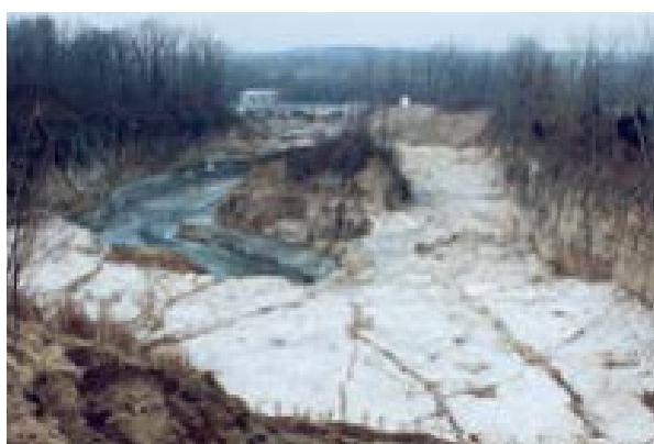
Figure 3: The quarry area during waste removal efforts prior to backfilling.
