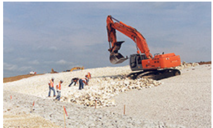
Figure 10: Consolidation of waste materials in the disposal cell (left). Workers placing the exterior cobble layer of the cover on the disposal cell (right).
