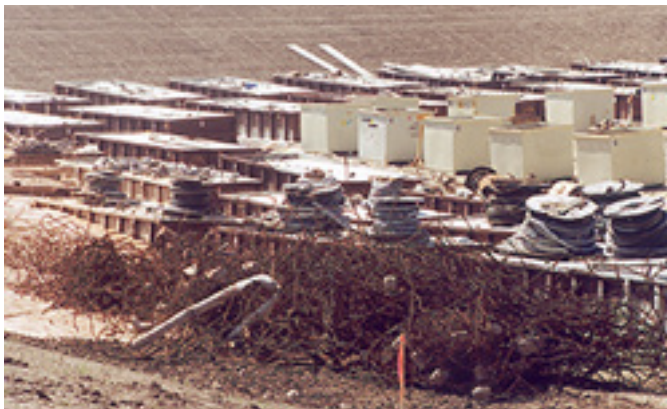
Figure 10: Consolidation of waste materials in the disposal cell (left). Workers placing the exterior cobble layer of the cover on the disposal cell (right).
