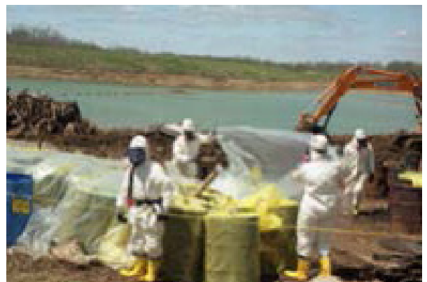
Figure 4: Removing abandoned materials for processing.
