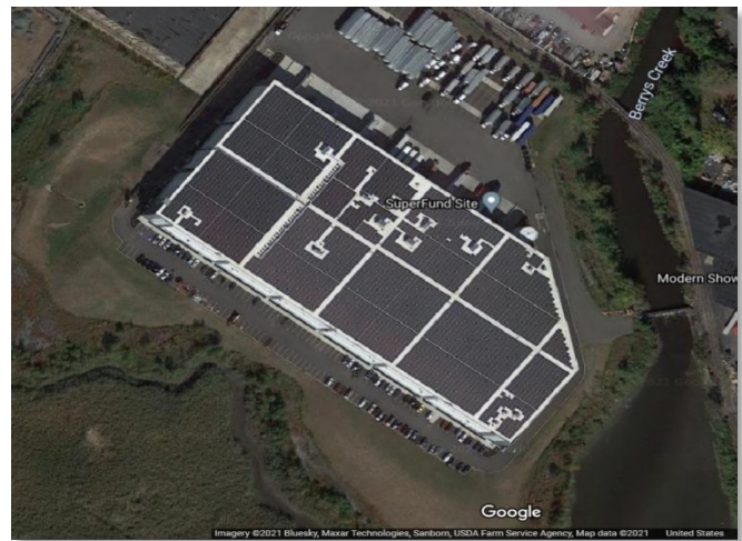
Figure 13. The solar array on the Duke Realty warehouse where Grace Kennedy and Mane Concept, Inc. operate.
