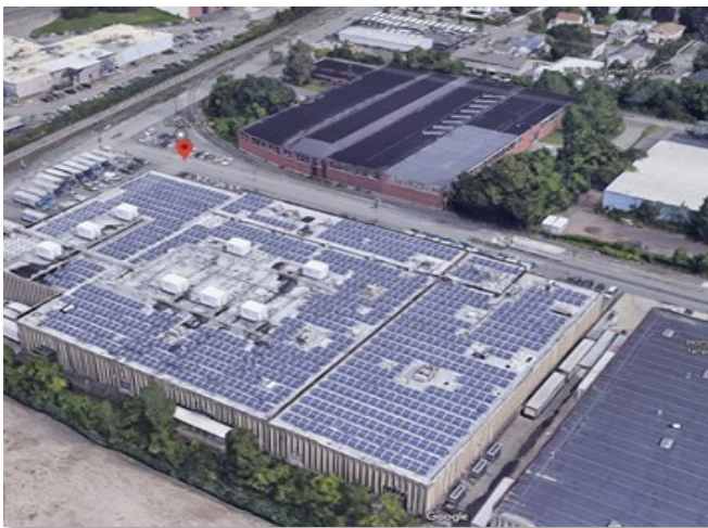
Figure 12. Solar arrays on Reddy Raw, Inc. (foreground) and Julius Blum & Co., Inc. (background).
