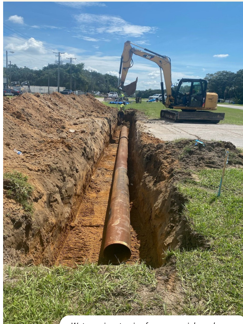
Water main extension for commercial supply
