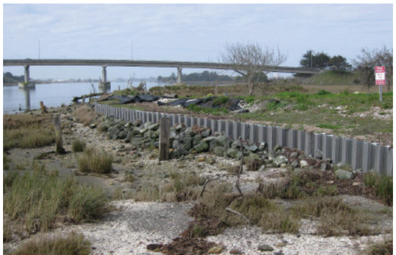
Figure 8. Protective measures for erosion control at the Tuluwat site (California).
