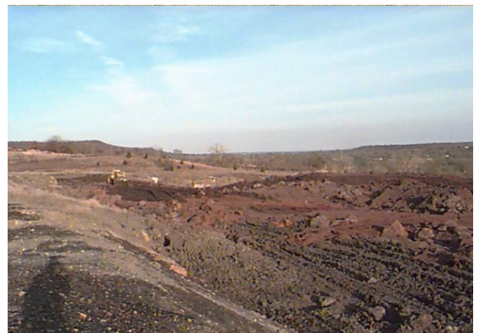
Contouring of site slag piles during cleanup. (Source: ODEQ)
