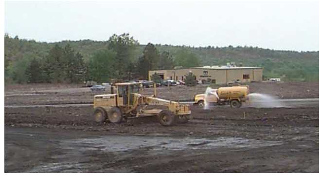
Final site grading. (Source: ODEQ)
