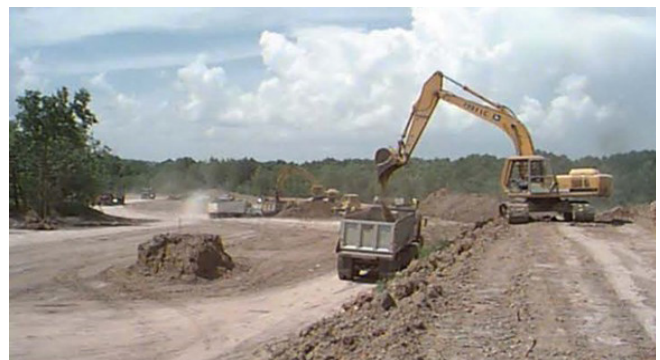
A nearby mining company donated overburden soil from its property to use as part of the site cap. (Source: ODEQ)
