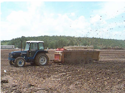
Cover soil placement. (Source: ODEQ)
