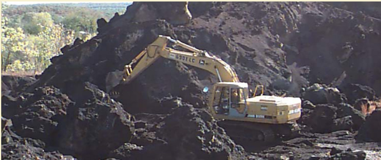
Slag pile cleanup on site. (Source: ODEQ)
