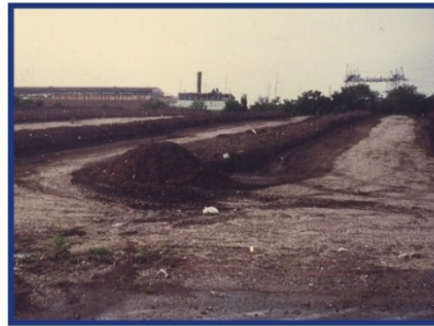
Before: Former landfill, including a former leaf compost area (above).
