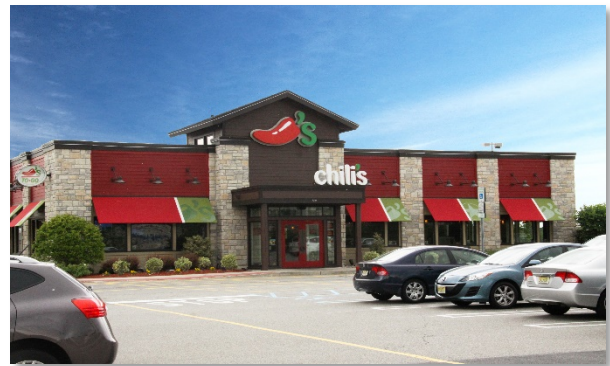
Figure 14. The Chili's restaurant on site.
