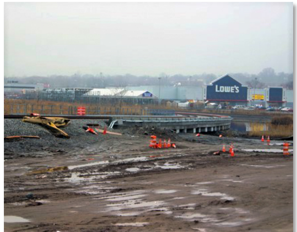
Figure 7. Rail line construction, April 2009 (Source: NJSEA).
