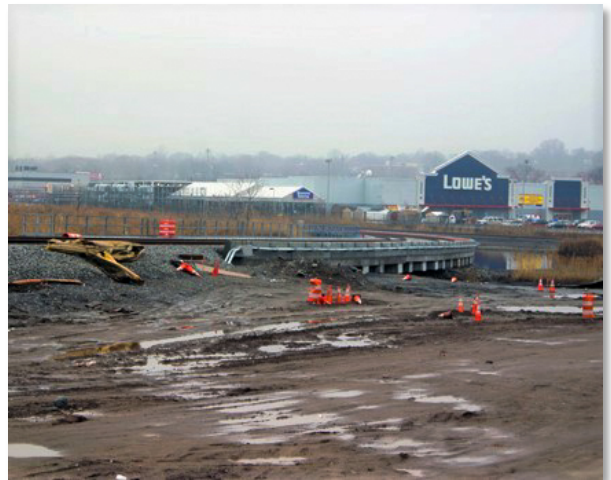
Figure 7. Rail line construction, April 2009 (Source: NJSEA).
