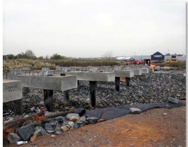
Figure 6. Rail line construction, October 2007 (Source: NJSEA).
