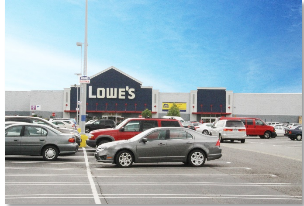
Figure 13. The Lowe's home improvement store on site.
