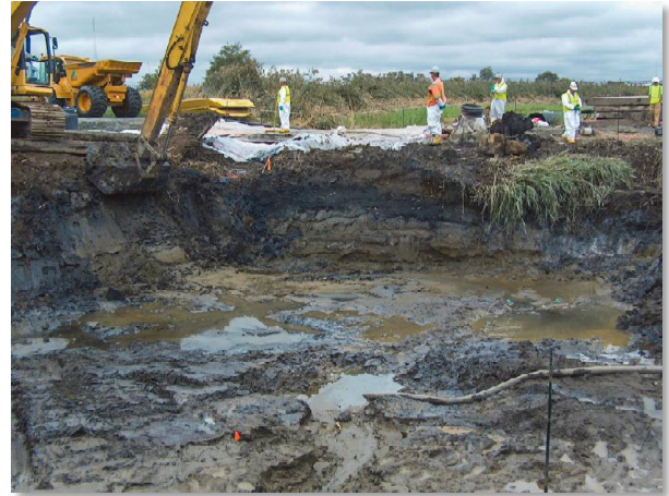
Figure 3. Excavation activities (Source: Honeywell International).
