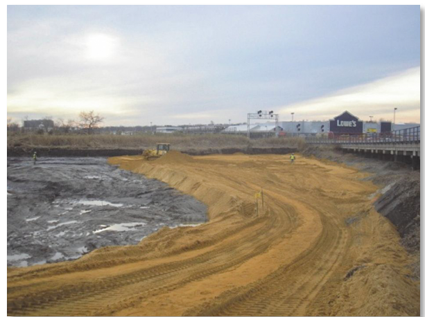
Figure 4. Start of backfill process (Source: Honeywell International)
