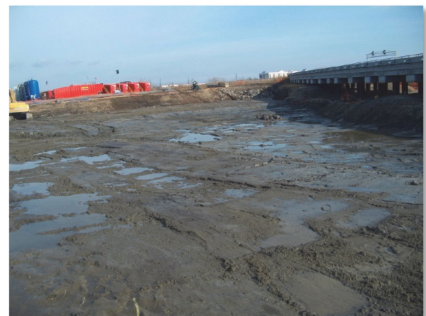
Figure 5. Excavation work at the lagoon (Source: Honeywell International).
