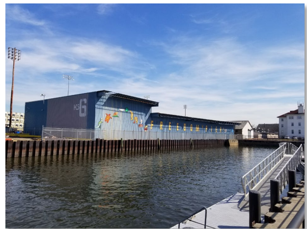
Figure 3. Port infrastructure at the Gloucester Marine Terminal today.
