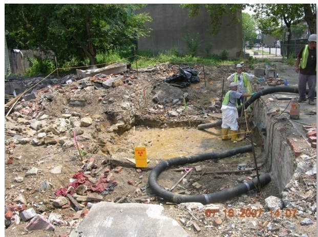
Figure 5. Excavation of a contaminated site property.
