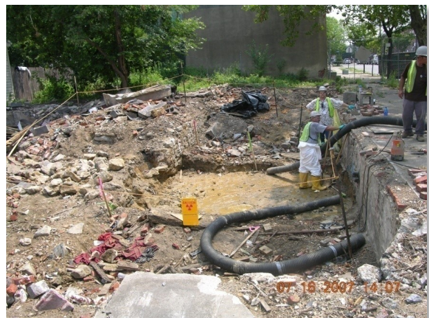
Figure 5. Excavation of a contaminated site property.
