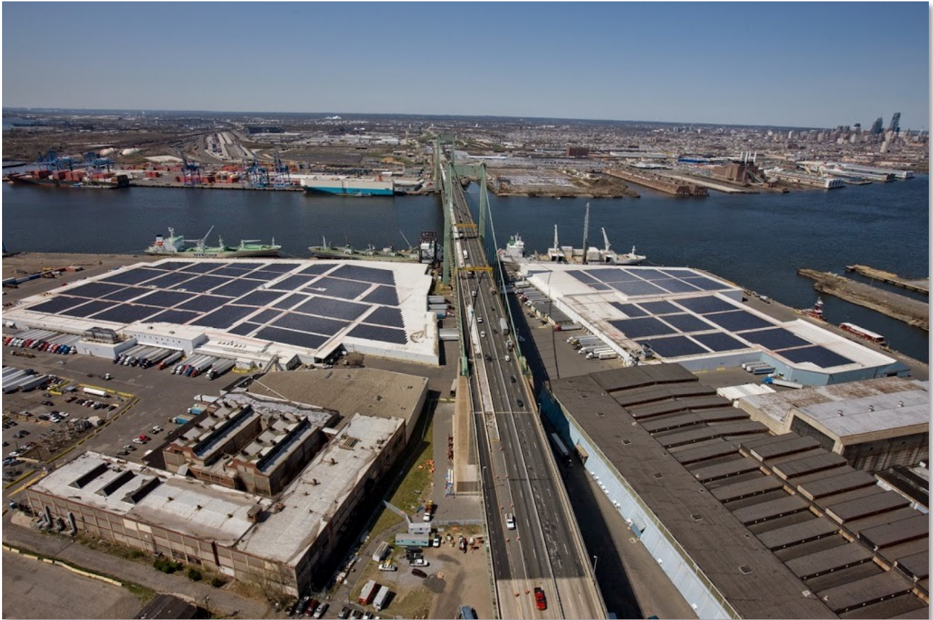
Figure 20. Aerial view of the Gloucester Marine Terminal and Walt Whitman Bridge (image used with permission of Holt Logistics Corp.).
