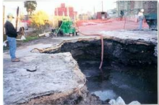
Figure 4. Removal of subsurface contaminants from 360 Concord Street.
