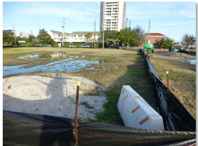
Figure 38. Additional site development underway.
