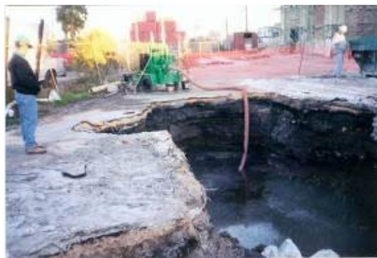
Figure 4. Removal of subsurface contaminants from 360 Concord Street.
