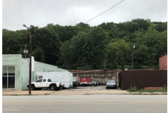
The parking lot at the Southwest Plating Co., Inc. site.
