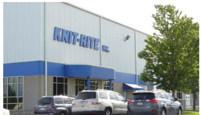
Business operating at the Osage Metal Company site.
