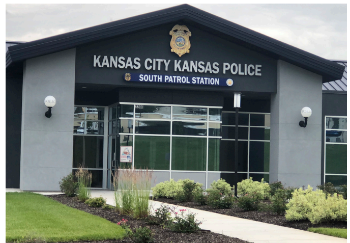
Land uses at the Kansas City Structural Steel site.
