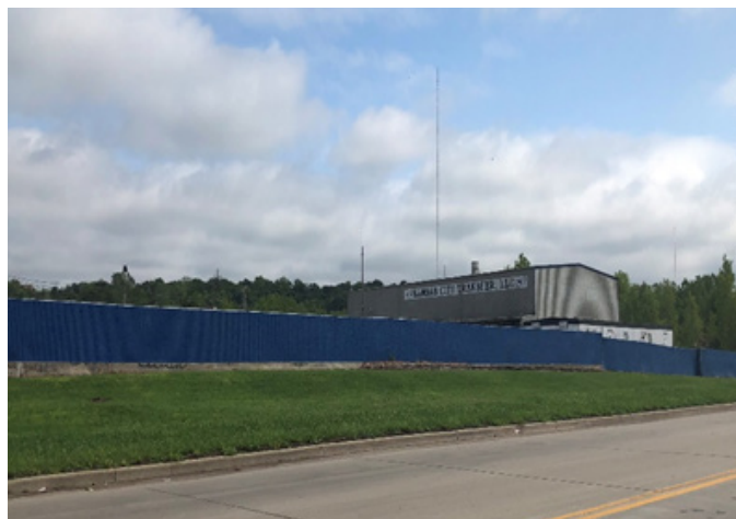
View of WCA Kansas City Transfer, LLC's facilities at the site.
