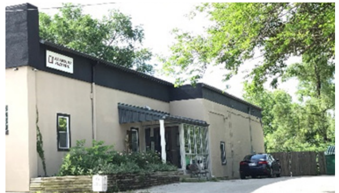
The electric repair company operating at the Kantex-KCMO site.
