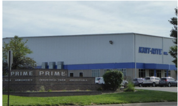
The main entrance to Knit-Rite Inc.'s facilities at the Osage Metal Company site.
