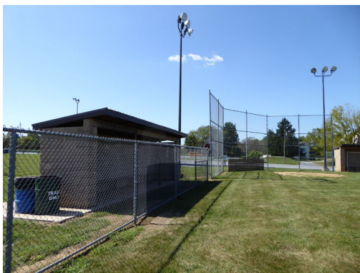
Figure 7. Jackson Recreational Park has a lighted baseball/softball field with aboveground dugouts.
