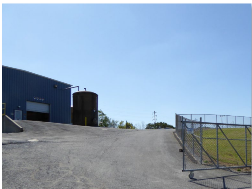
Figure 3. Groundwater cleanup takes place at the site's groundwater treatment facility.
