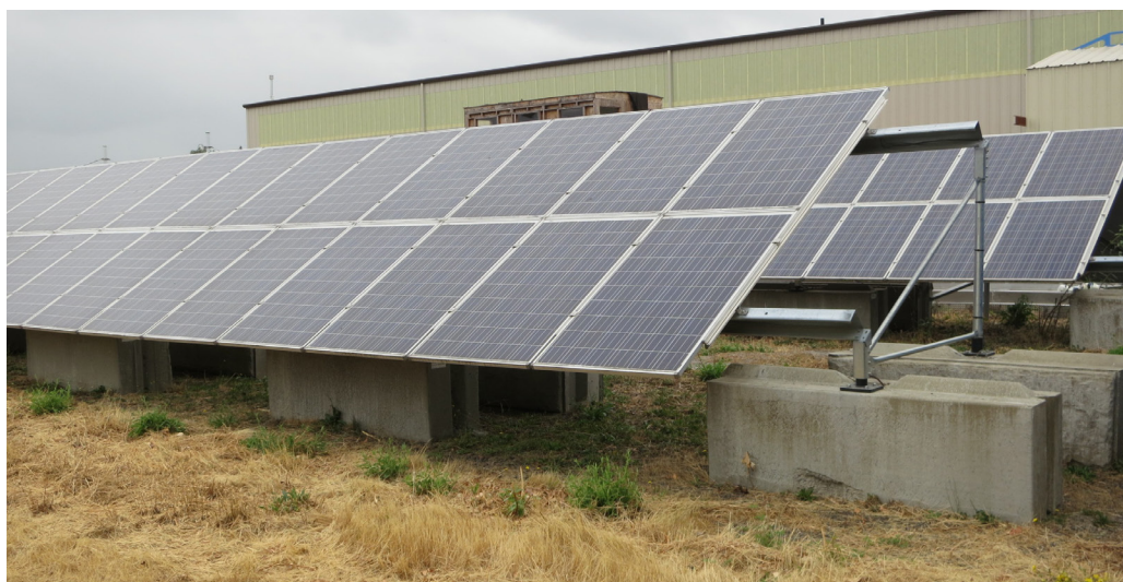
Figure 13. Solar installation at the Northwest Pipe & Casing/Hall Process Company Superfund site (Oregon).
