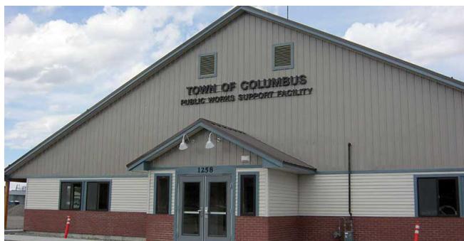
Figure 20. The town of Columbus' public works building at the Mouat Industries site.
