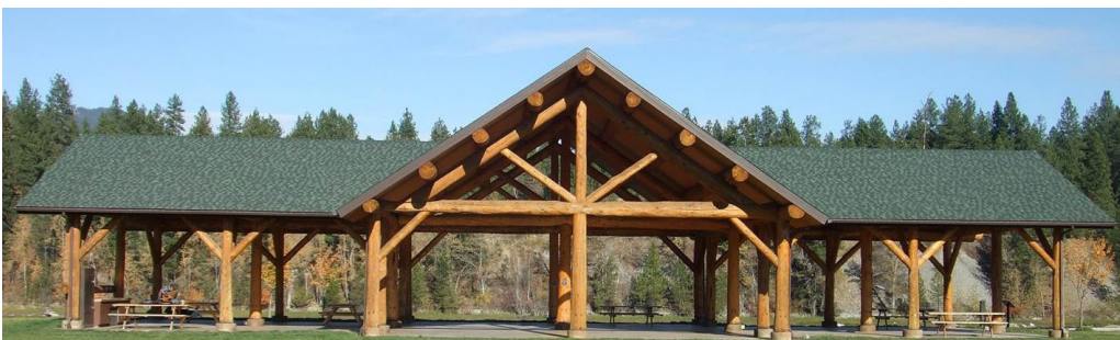
Figure 15. The Fred Brown Riverfront Pavilion at the Libby Asbestos site (Montana).
