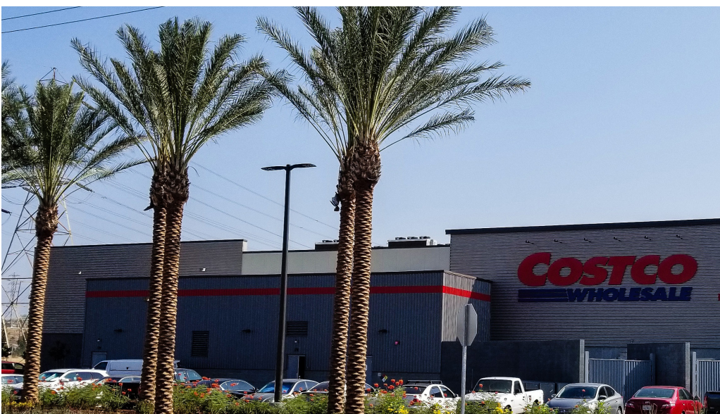
Figure 13. The new Costco store at the Operating Industries, Inc., Landfill site (California).
