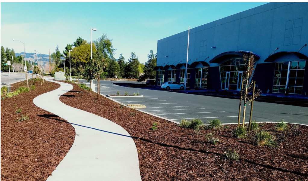
Figure 12. The Cader Corporate Center and a walking path at the Sola Optical USA, Inc. site (California).
