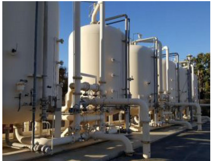
Figure 10. Tanks used in treating groundwater at the Newmark Ground Water Contamination site (California).
