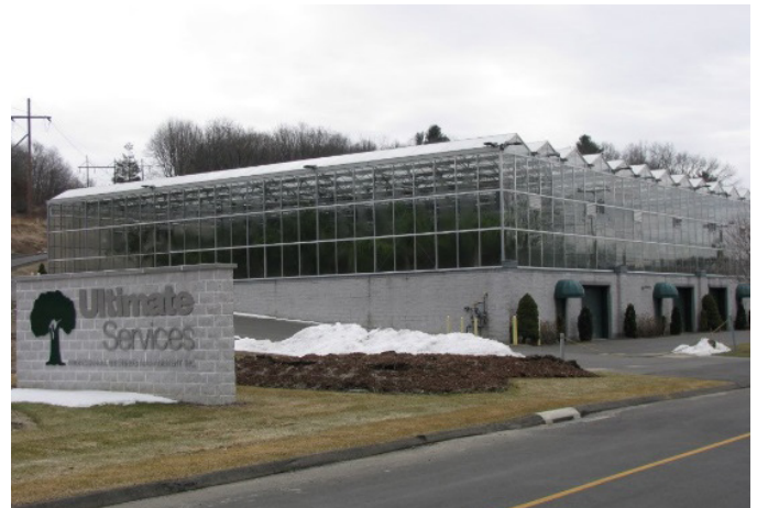
Figure 42. New building at the Nutmeg Valley Road site (Connecticut).
