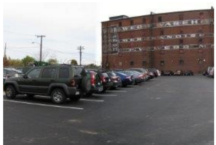
Figure 89. Parking and warehouse facilities at the Universal Steel & Trading Corporation site (Massachusetts).
