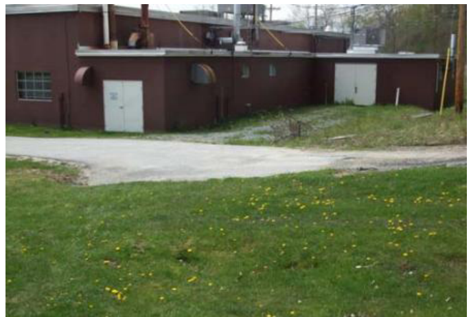
Figure 112. Facilities at the Tansitor Electronics, Inc. site (Vermont).
