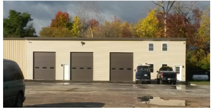
Figure 92. Facilities in reuse at the Kearsarge Metallurgical Corp. site (New Hampshire).
