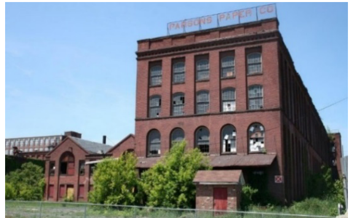
Figure 87. View of the Parsons Paper site (Massachusetts).
