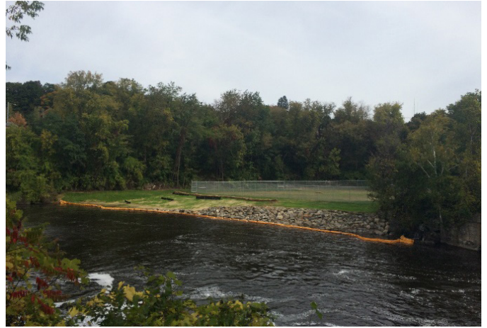
Figure 100. View of the former Synergy Site (New Hampshire).
