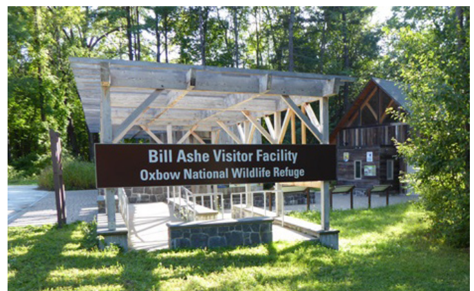
Figure 75. The Bill Ashe Visitor Facility at the Fort Devens site (Massachusetts).
