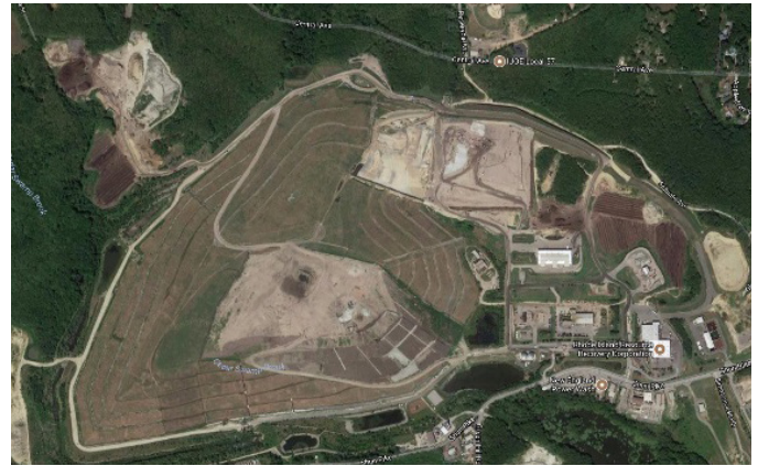
Figure 101. Aerial view of the Central Landfill site (Rhode Island). Imagery © 2017 Google.
