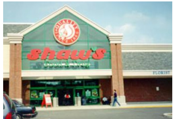
Figure 58. Entrance to the Shaw's Supermarket at the Bangor Gas Works site (Maine).
