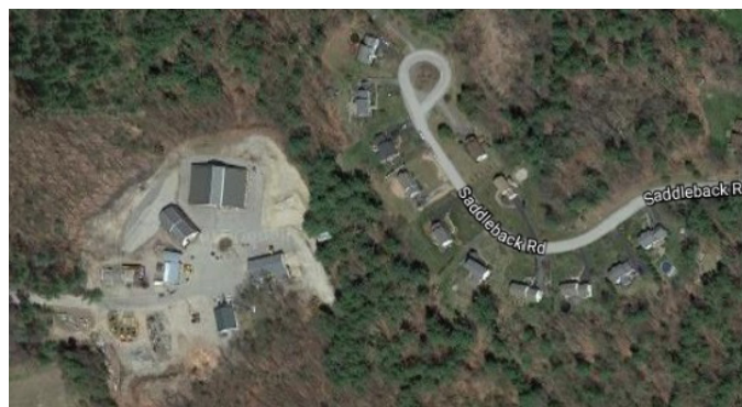
Figure 97. Residential development east of the Town Garage/Radio Beacon site (New Hampshire). Imagery © 2017 Google.
