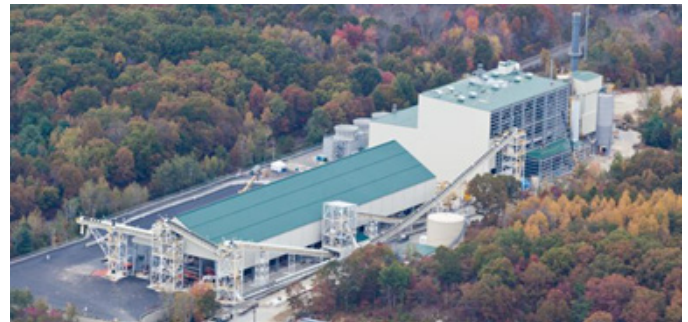
Figure 40. The Greenleaf biomass facility at the Gallup's Quarry site (Connecticut). Image used with permission of Greenleaf Power LLC.
