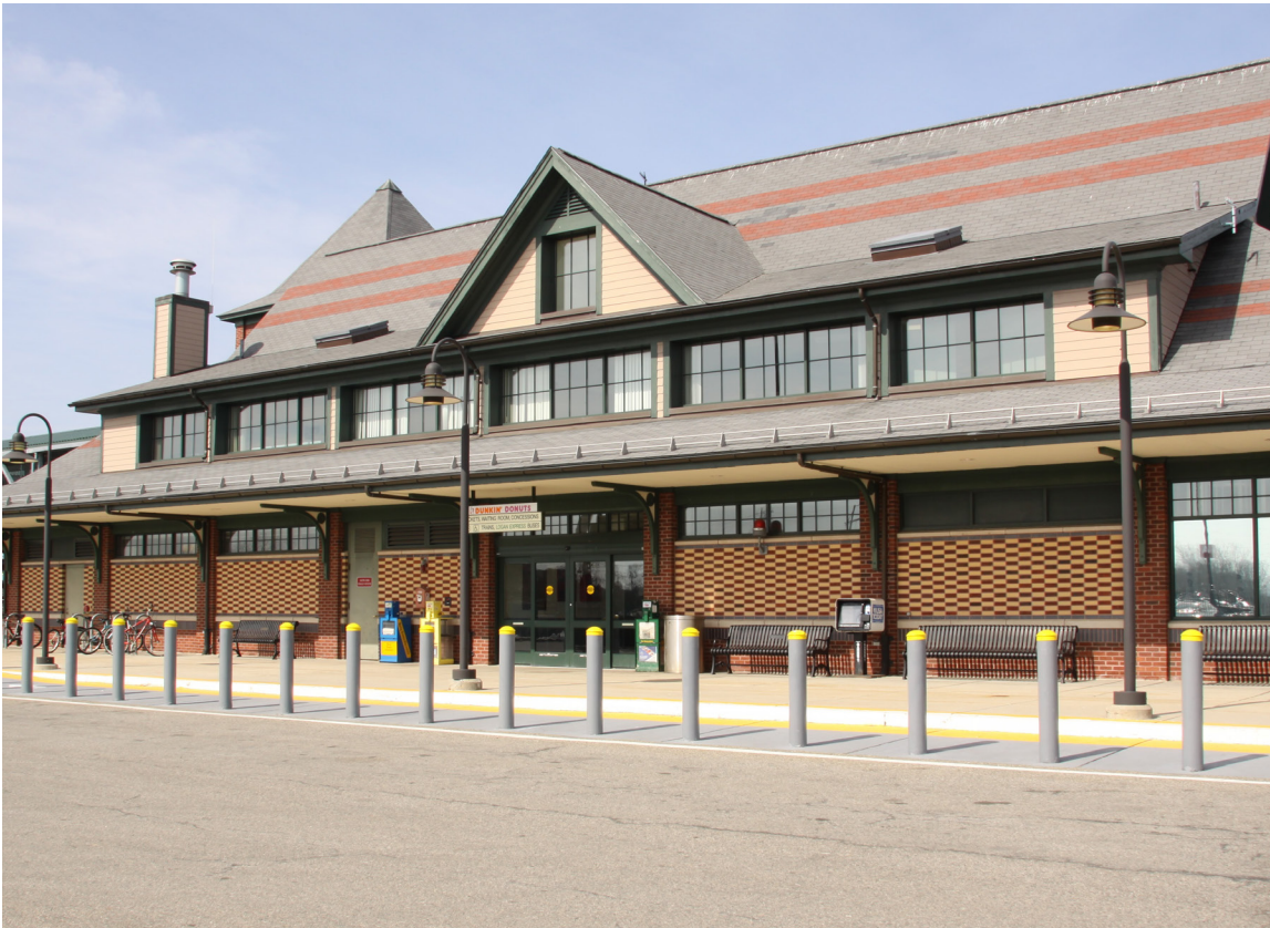
Figure 1. The James Anderson Regional Transportation Center opened at the Industri-Plex site in 2001 (Massachusetts).
