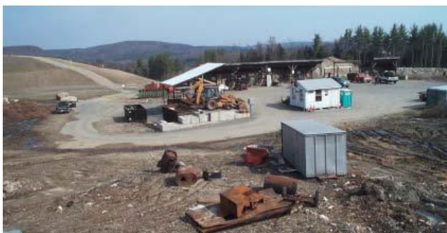
Figure 31. Recycling center at the Barkhamsted-New Hartford Landfill site.
