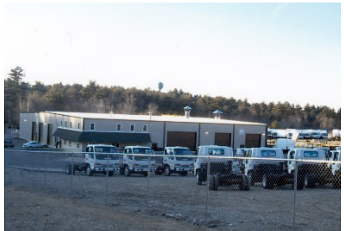
Figure 106. View of the Western Sand & Gravel site (Rhode Island).
