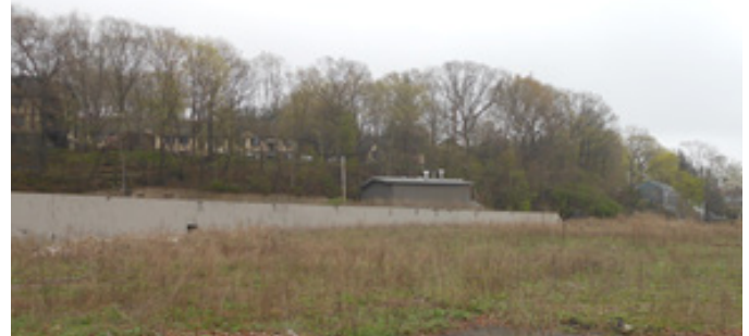
Figure 41. Commercial space and groundwater treatment building at the Kellogg-Deering Well Field site (Connecticut).
