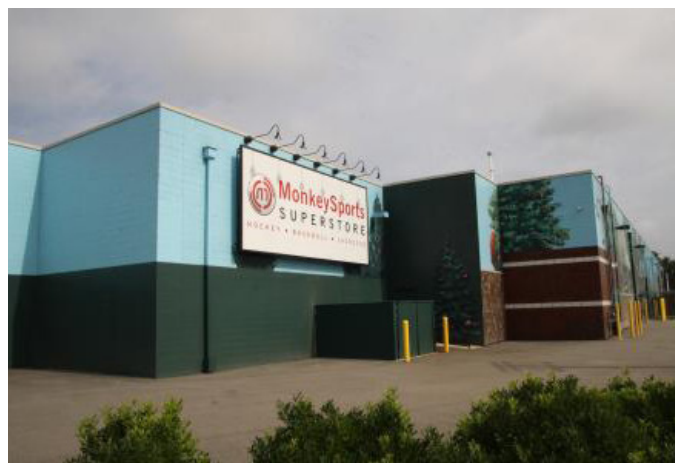
Figure 68. Commercial facilities at the Norwood PCBs site (Massachusetts).
