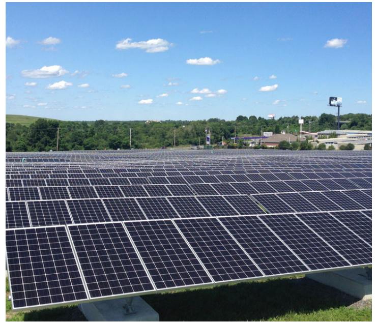
Figure 5. Over 5,000 block-mounted, fixed-tilt solar panels are in operation at the Sullivan’s Ledge site (Massachusetts).
