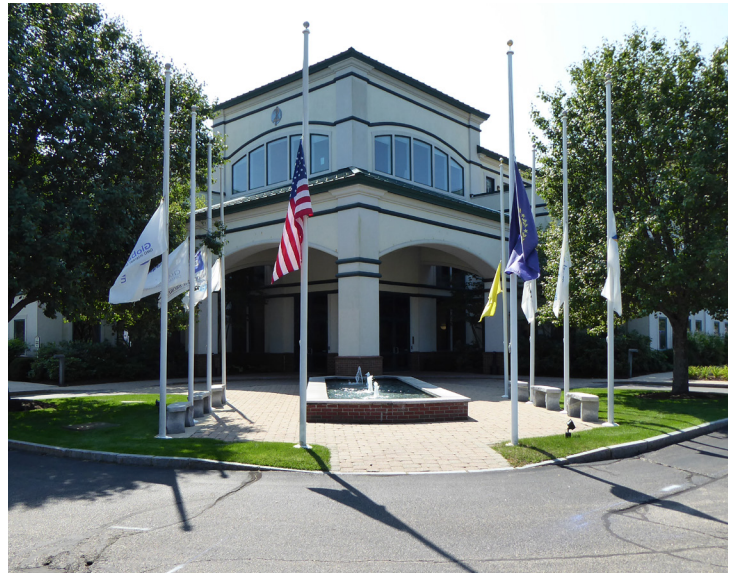
Figure 14. Businesses at the Pease Air Force Base site (New Hampshire).
