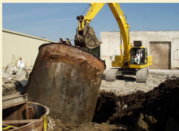
Removal of an underground mixing vat.
