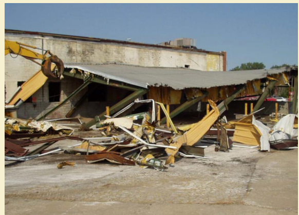
HABCO building demolition.
