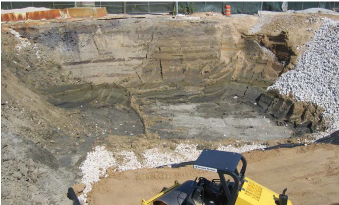
Phase 2 removal excavation along Railroad Avenue.
