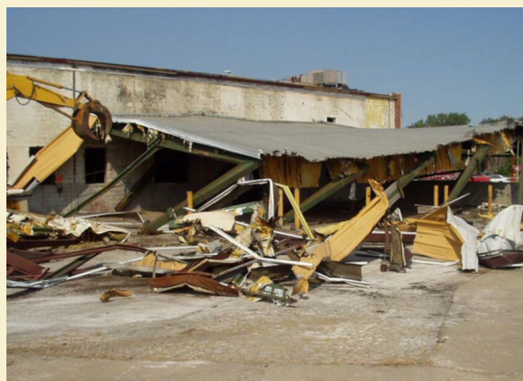
HABCO building demolition.
