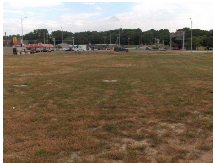
Gravel cover over an area of excavation at the end of phase 1 of the removal action in 2004 (left) and vegetated cover over an area of excavation at the end of phase 2 of the removal action in 2006 (right).
