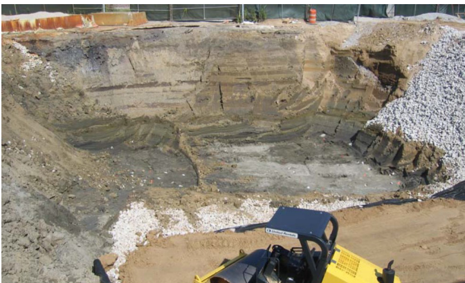
Phase 2 removal excavation along Railroad Avenue.
