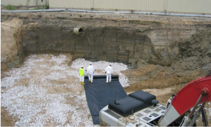
Phase 2 removal excavation up to the wall of the hardware store next to the site.
