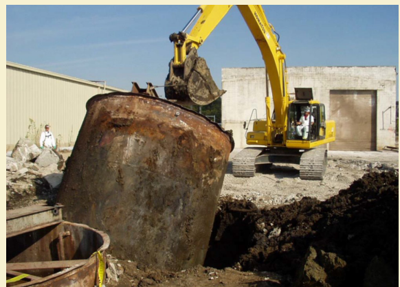
Removal of an underground mixing vat.
