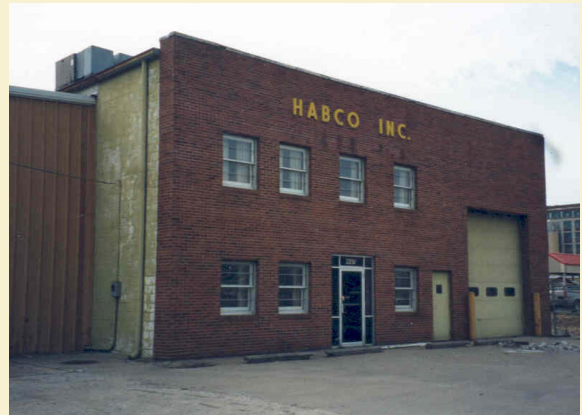
Former HABCO building before demolition.
