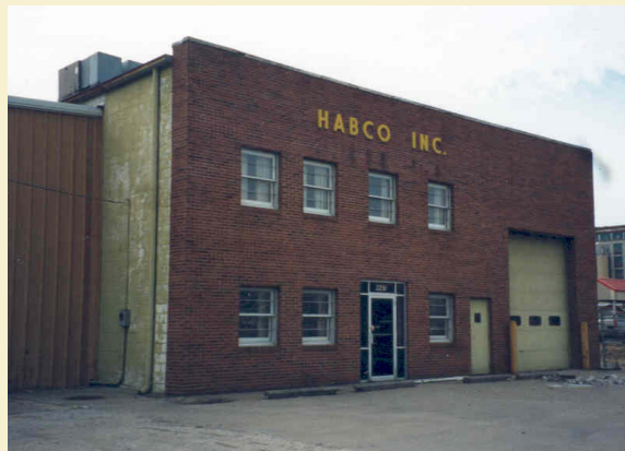
Former HABCO building before demolition.
