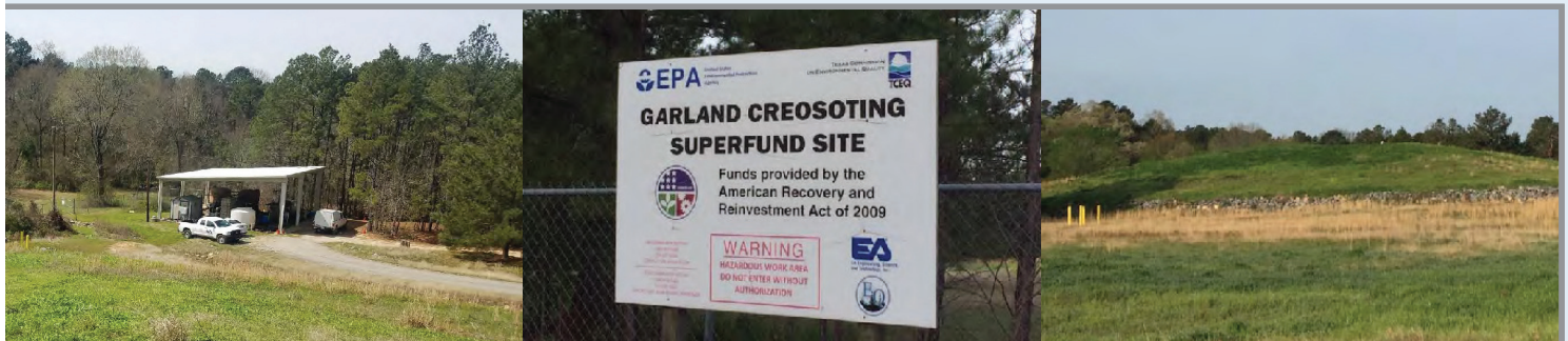
Images from left to right: Groundwater treatment plant, sign at entrance to site, and view of the on-site soil repository.
