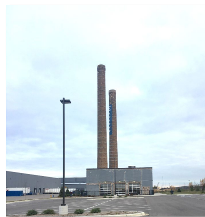
Figure 5. The former NIROP smokestacks that serve as inspiration for Northern Stacks Industrial Park.
