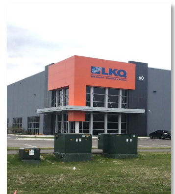
Figure 15. LKQ's location at Northern Stacks.
