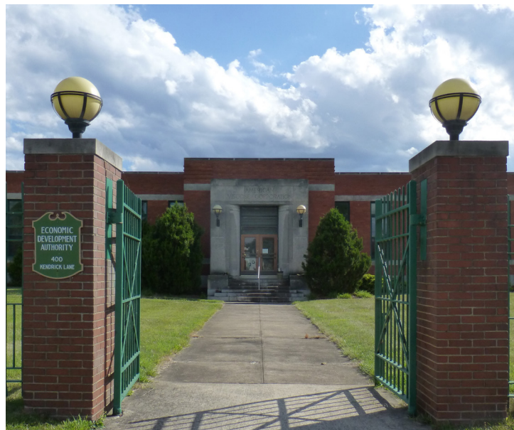
Figure 15. The former American Viscose Corporation administrative building now houses several small businesses and the Front Royal-Warren County Economic Development Authority at the Avtex Fibers, Inc. site (Virginia).
