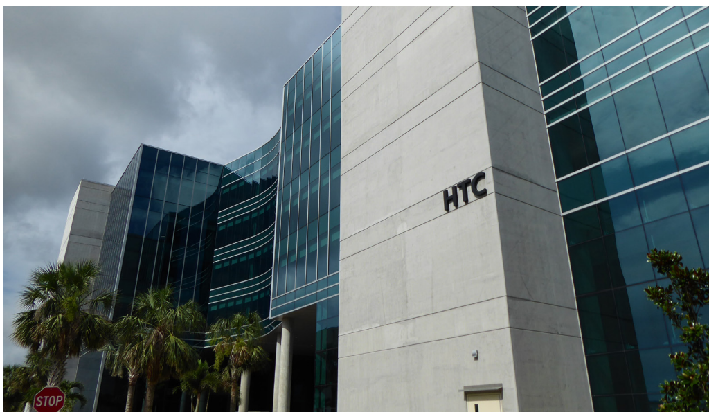
Figure 10. The Harris Technology Center at the Harris Corp. (Palm Bay Plant) site (Florida).
