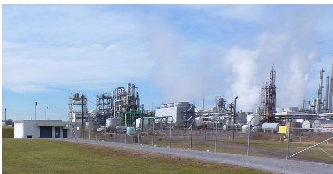
Figure 19. Ongoing chemical manufacturing at the B.F. Goodrich site.
