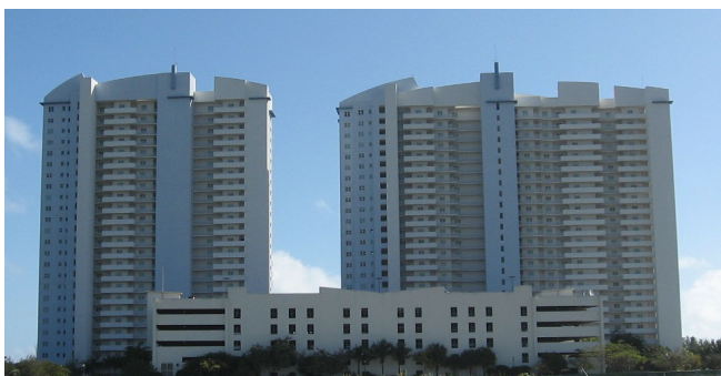
Figure 17. The two residential towers at the Munisport Landfill site.
