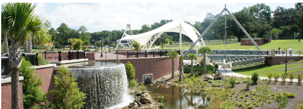
Figure 12. Cascades Park and the Capital City Amphitheater at the Cascade Park Gasification Plant site (Florida). Image used with permission of the city of Tallahassee.
