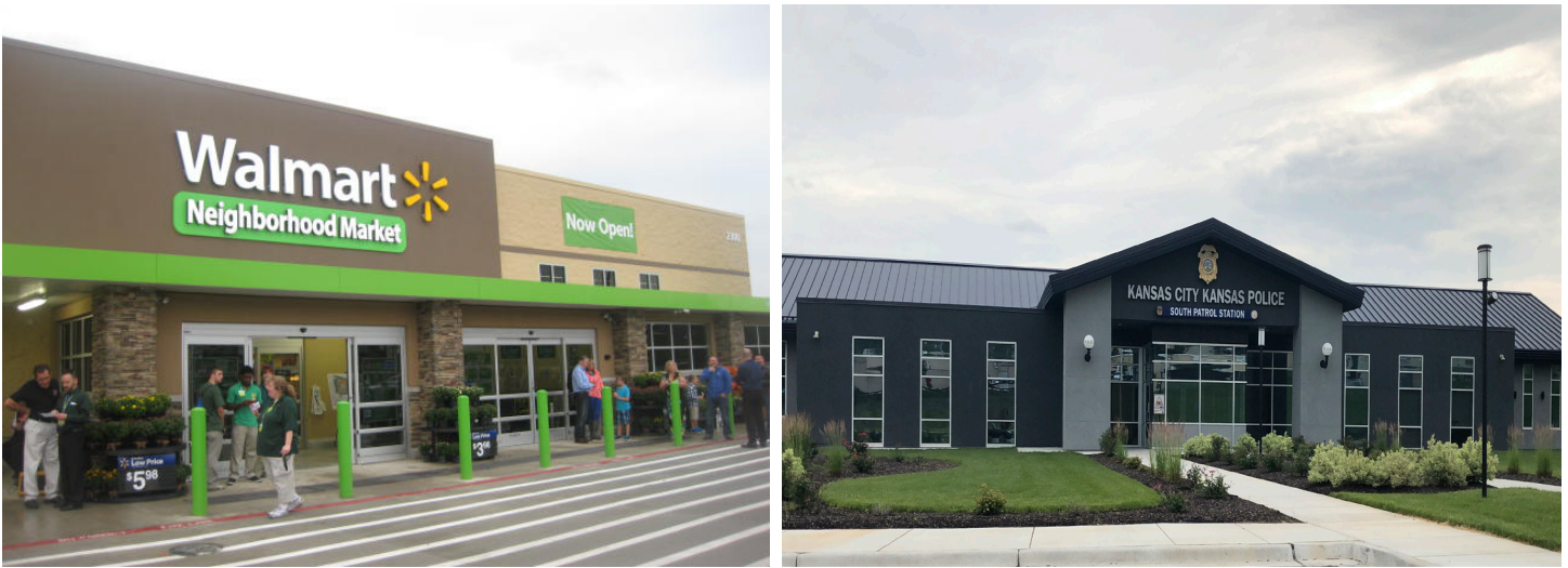
Figure 6. Left: Walmart Neighborhood Market at the Kansas City Structural Steel site (Kansas). Right: The new police station at the Kansas City Structural Steel site (Kansas).
