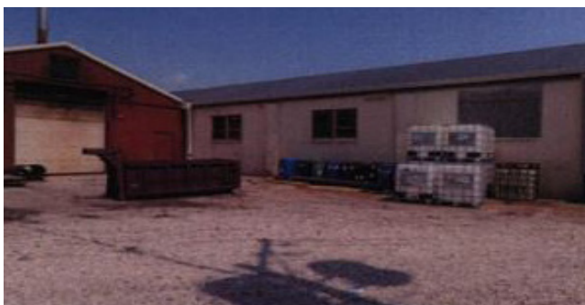
Figure 15. This metal-plating facility continues to operate at the Electro-Coatings, Inc. site.
