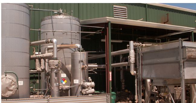
Figure 23. The award-winning gas-to-liquid fuel technology demonstration project.
