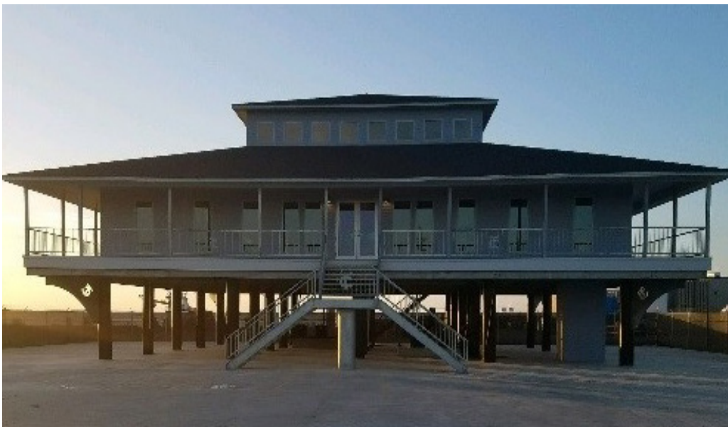
Figure 15. Tubal-Cain headquarters at the Palmer Barge line site (Texas).
