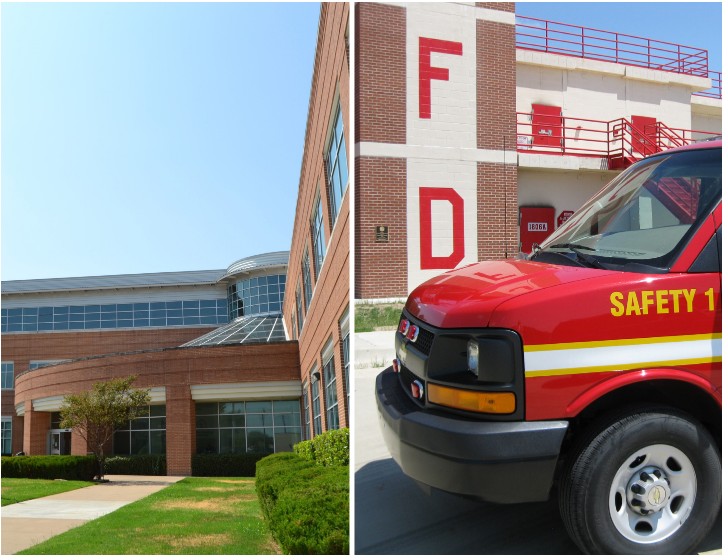
Figure 3. Left: The Dallas Housing Authority Central Office at the RSR Corporation site (Texas). Right: The four-story burn tower at the Vertac, Inc. site provides firefighter and police response training (Arkansas).
