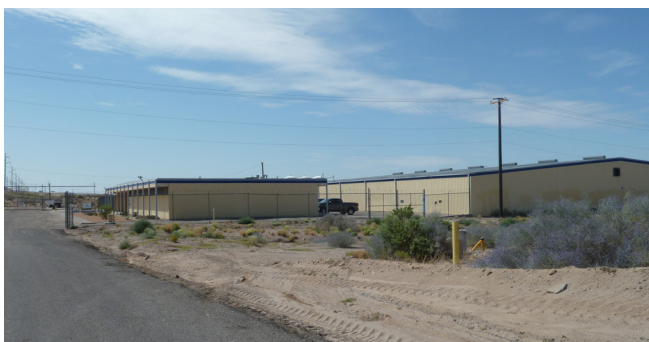
Figure 22. Univar USA continues to operate at the South Valley site.
