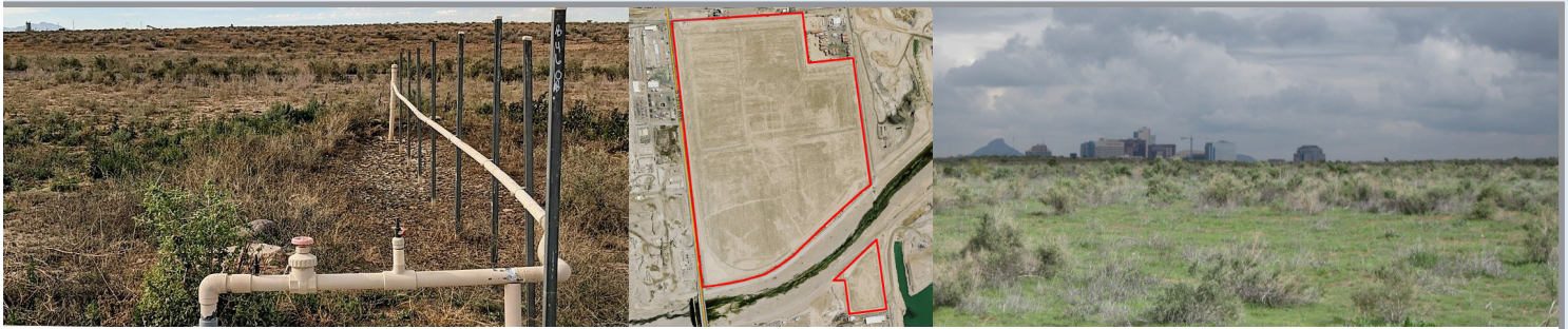
Images from left to right: View of the gas extraction system; Aerial view of the site; View of the landfill cap looking northeast toward downtown Phoenix.
