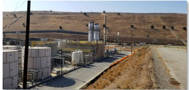
Figure 3. The on-site leachate treatment plant operated by New Cure, INC.
