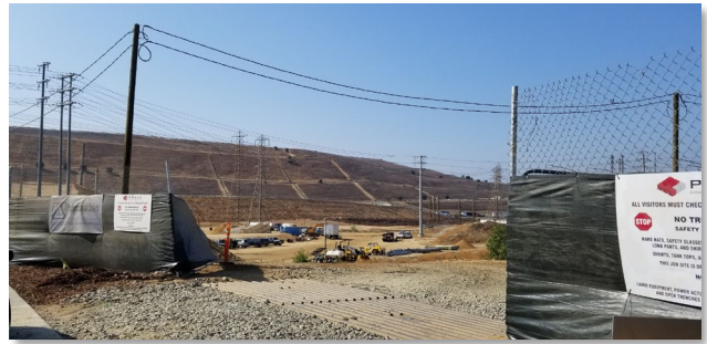
Figure 4. Redevelopment construction at the site, August 2018.
