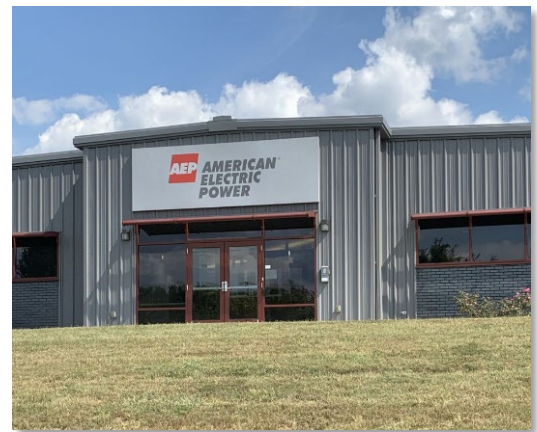
Figure 8. American Electric Power's facility on site.
