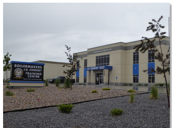
Figure 10. The WSJAC J.G. Cooksey Training Center provides training services for aspiring boilermakers.
