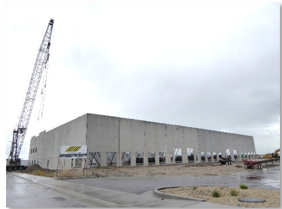
Figure 12. New construction at the site.
