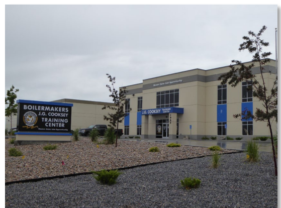
Figure 10. The WSJAC J.G. Cooksey Training Center provides training services for aspiring boilermakers.
