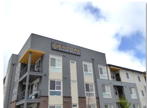
Figure 10. The recently constructed Encore Evans Station on site.
