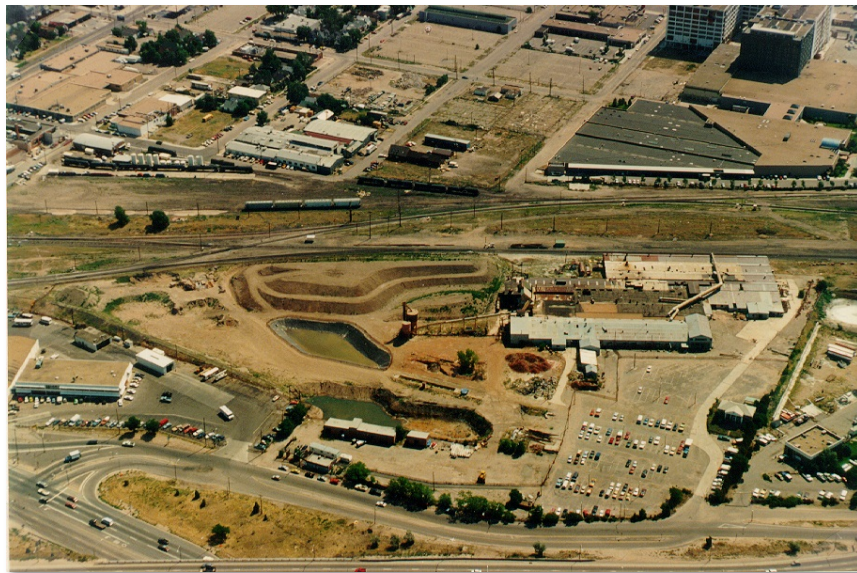
Figure 12. An aerial view of OU4/9B when Home Depot was under construction.
