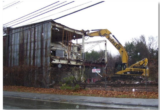
Figure 6. Demolition of dilapidated buildings before cleanup.
