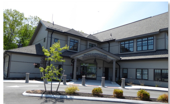
Figure 7. The entrance to the Walpole Co-operative Bank South Street Senior Center.
