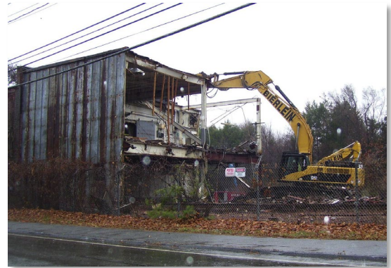
Figure 6. Demolition of dilapidated buildings before cleanup.
