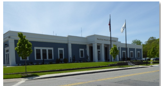
Figure 9. View of the front of the Walpole Police Department building on site.
