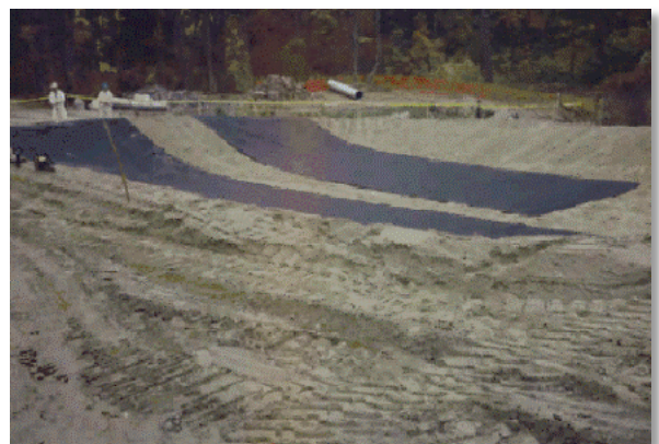
Figure 5. Cap installation following soil excavation.
