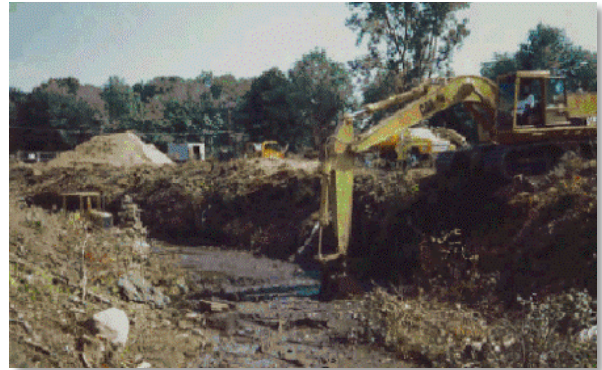
Figure 3. Cleanup included removal of asbestos contamination along the Neponset River.
