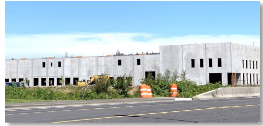
Figure 5. Development of a new lot underway at TRIP.
