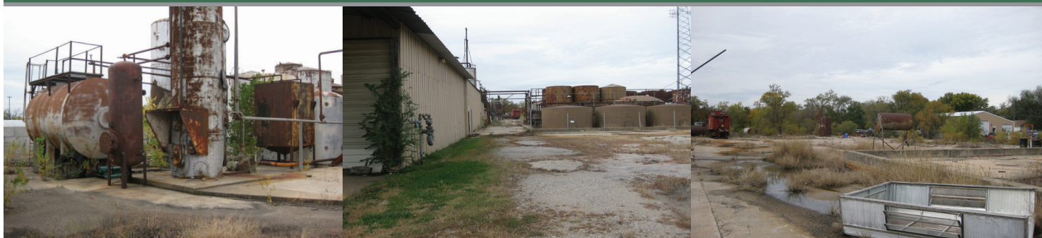
Images from left to right: View of storage tanks, infrastructure and wells at the Midland property.
