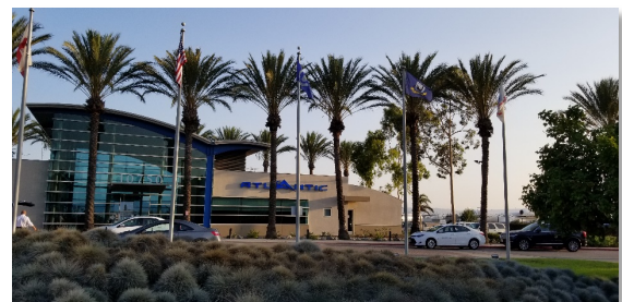
Figure 20. Atlantic Aviation's facility.
