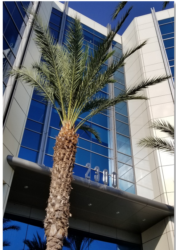
Figure 17. Cast & Crew offices.
