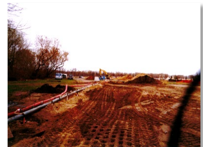
Figure 5. Dewatering operations in 1998. Source: MPCA.
