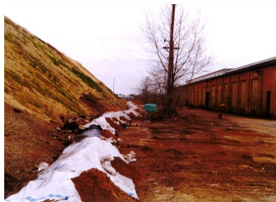
Figure 4. Looking east of the containment cell in 1998. Source: MPCA.
