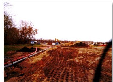
Figure 5. Dewatering operations in 1998. Source: MPCA.
