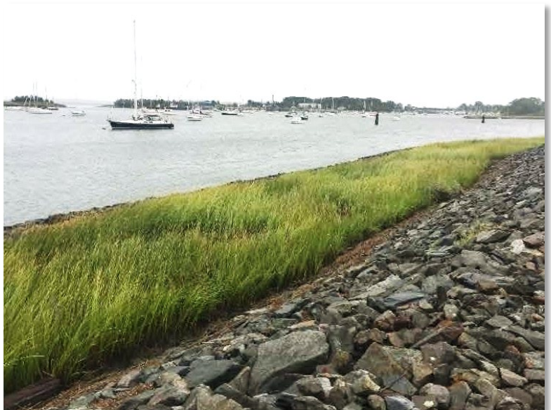
Figure 5. Current view of the revetment wall and wetland at Allen Harbor Landfill.
